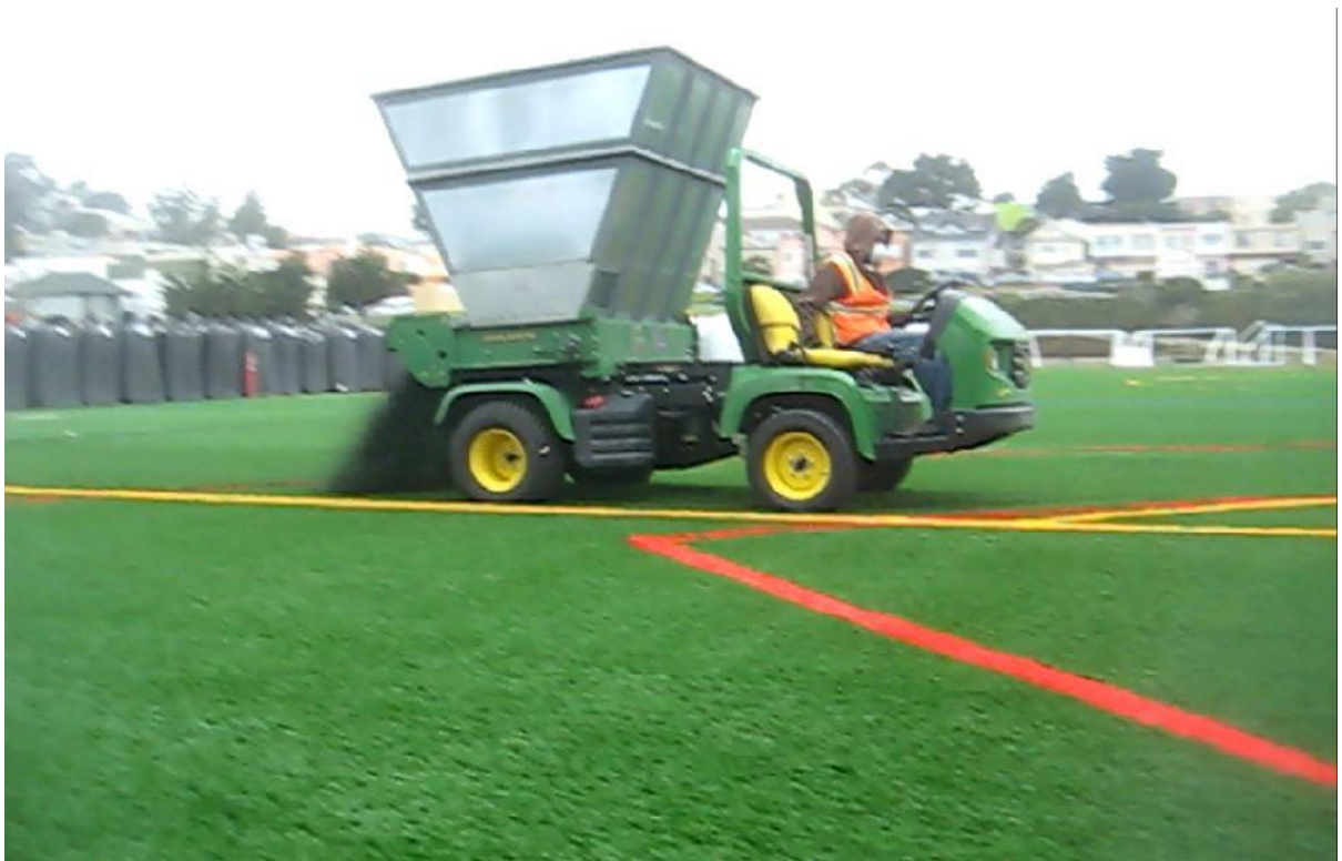
Figure A 9: Semi-mechanised application of infill
