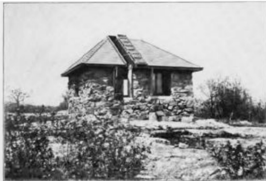
FIG. 1. — THE GEODETIC OBSERVATORY.
